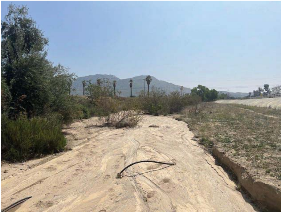
Photograph 11: South-facing view of channel in Reach 4 from Photo Point 11.
