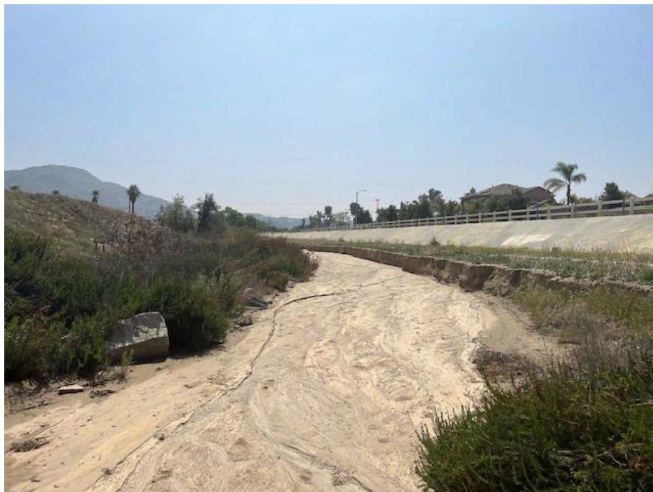
Photograph 10: South-facing view of channel at the southern boundary of Reach 3, looking into Reach 4 from Photo Point 10.
