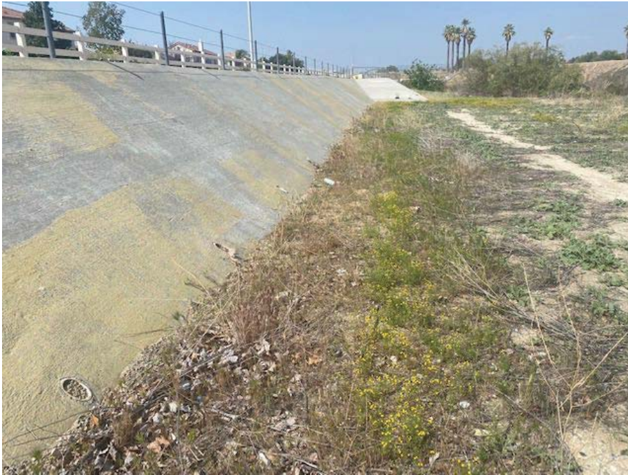
Photograph 31: Weep holes at the base of a concrete flood control wall on the west side of the channel.
