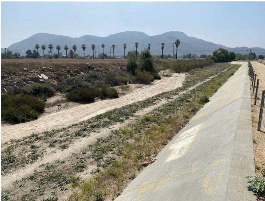
Photograph 20: Overview of Reach 4 and Reach 5 from Photo Point 20.
