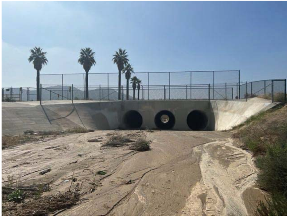
Photograph 1: South-facing view of Reach 1, from Photo Point 1, where three concrete-encased culverts pass under Cottonwood Avenue.
