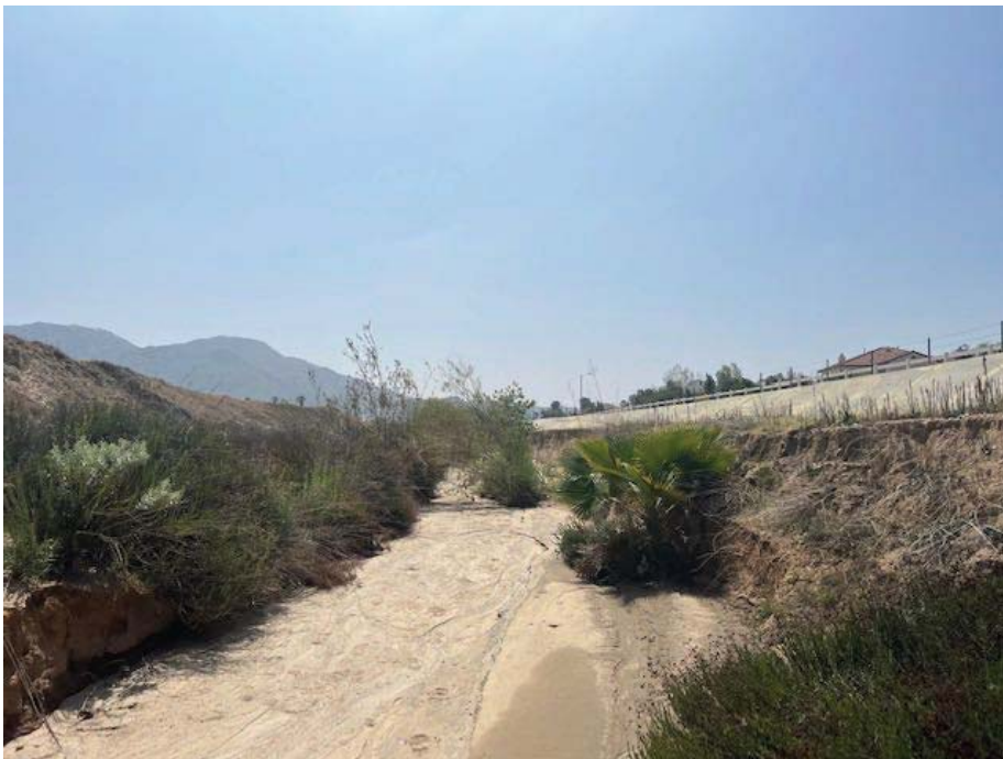
Photograph 4: South-facing view of channel in Reach 2 from Photo Point 4.
